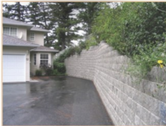
NEAR VERTICAL, COMPOSITE WALLS
