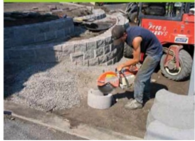
Precision cutting of blocks to shape
