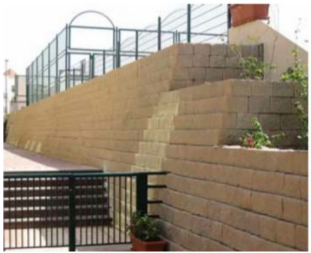
Precision cutting of blocks to shape
